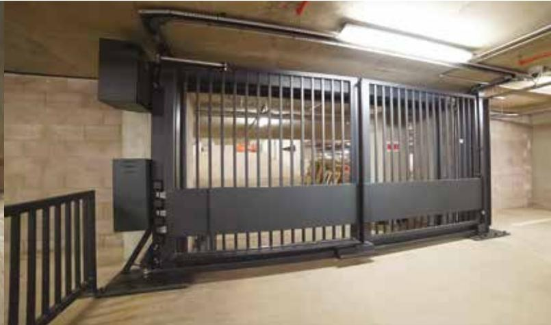
Cova Security Gates have worked with world leading HVM Security Specialists to design and deliver our first Engineered Solution Crash Rated 'Surface Fixed' 30mph (48km/h) Bi-Folding Gate - CSG 10630.
